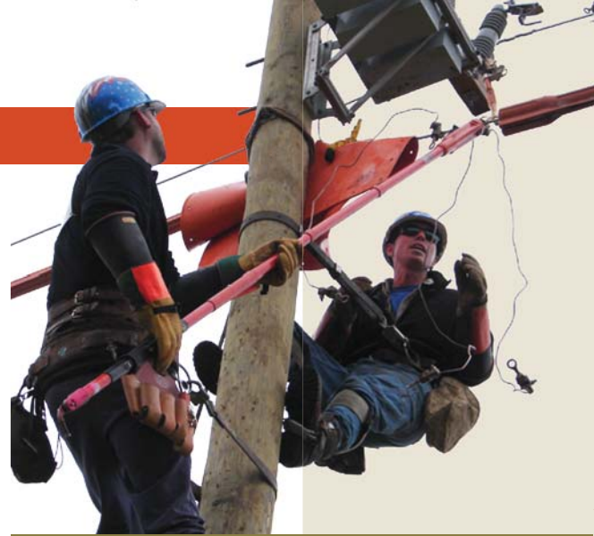
CVEC linemen T. R. Eubank and Larry Campbell competing at Rodeo in the "Capacitor Change-out" event.
